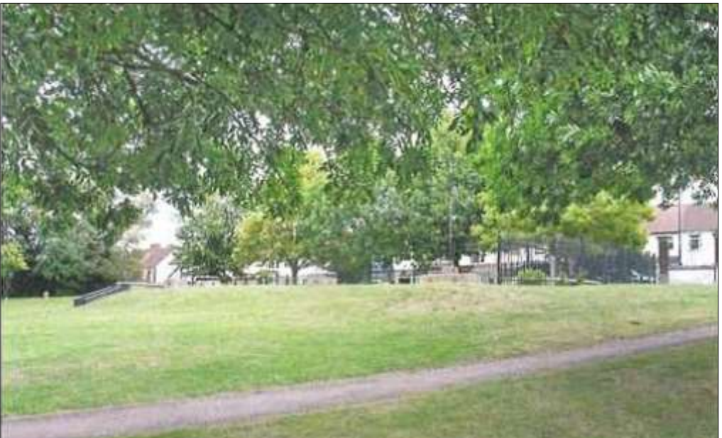
The outside of the bunker viewed from within Woodlands Park
