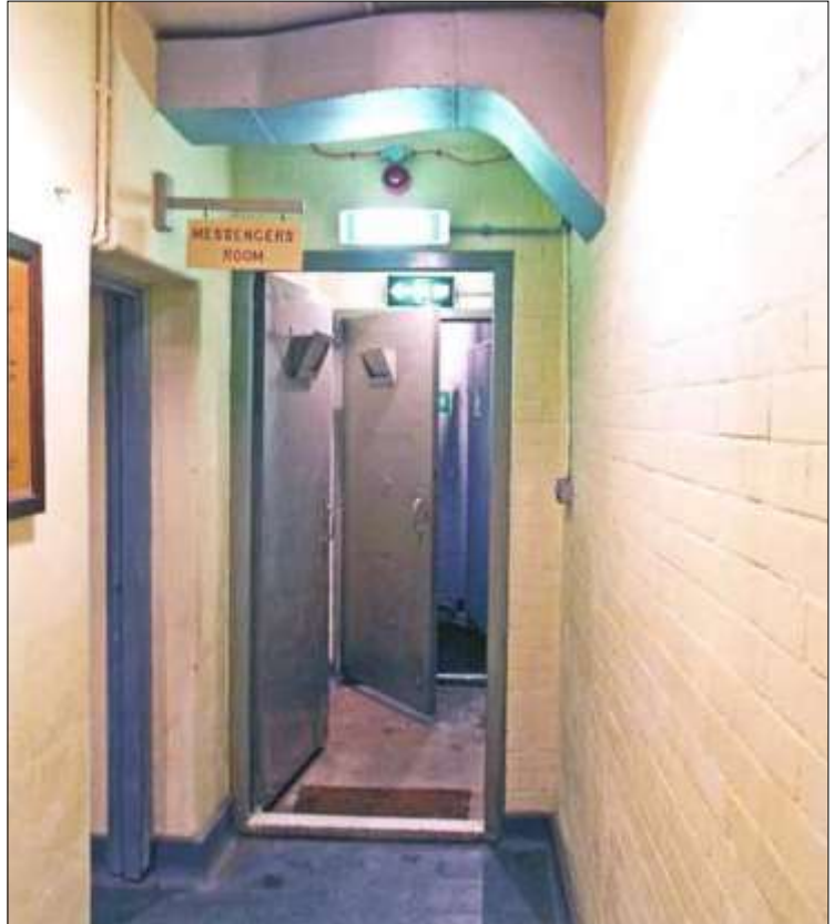
Spine corridor looking back towards the entrance doors with their flapped apertures.
