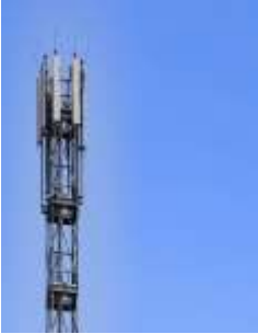
A cell tower
