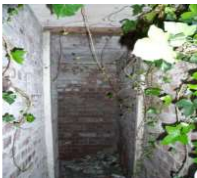
The entrance to ARP Wardens Post, Albermarle, Plymouth
